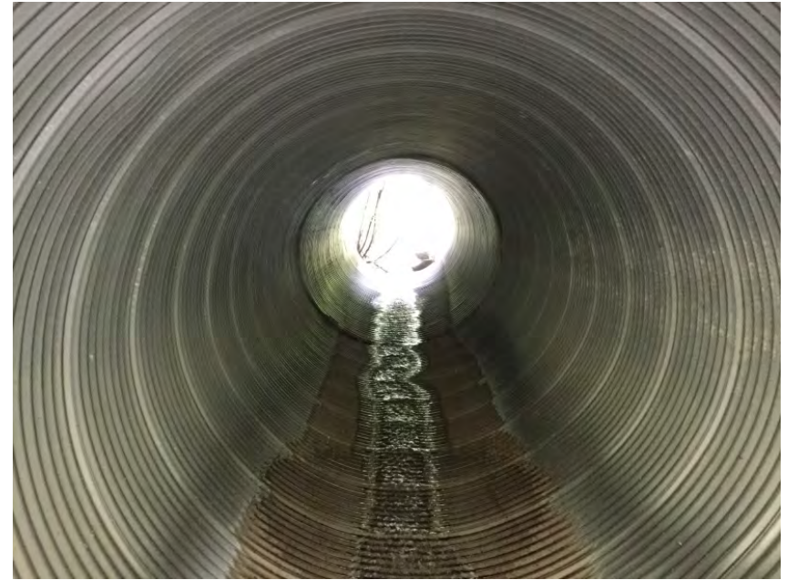
Looking through from inlet
